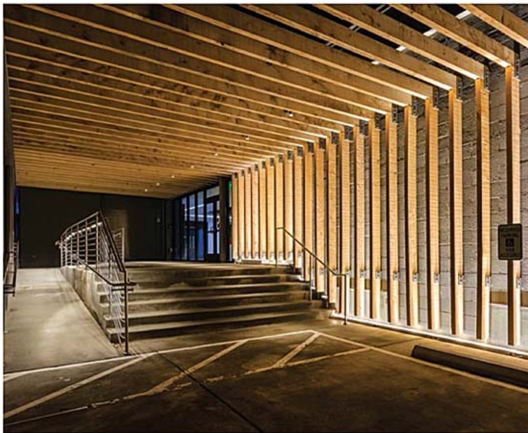
Colorful interior features are visible from outside, where low-level wall washers and in-grade LEDs forge a nighttime identity for the building.
